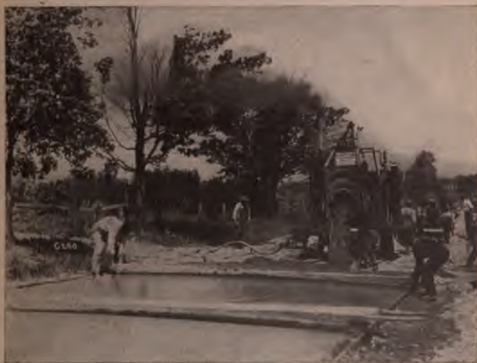
Chain-Belt Mixer on Milwaukee County Roads.
